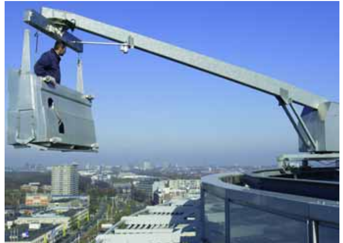
ANSI/IWCA I-14.1, sec. 5.7.12 states: “Rope descents shall not exceed 300 feet.” Therefore, buildings over 300 ft. are best suited with permanently installed powered platform .
