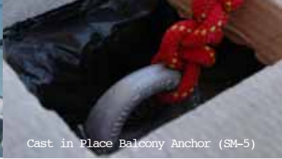
Cast in Place Balcony Anchor (SM-5)
