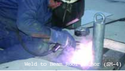
Weld to Beam Roof Anchor (SM-4)
