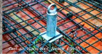
Cast in Place Roof Anchor (SM-5)
