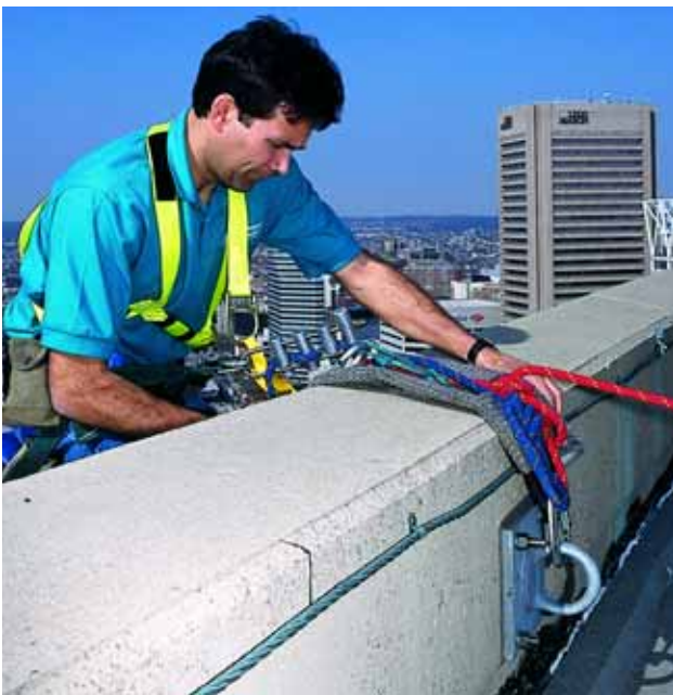
Parapet must be capable of supporting the load imposed by workers.
