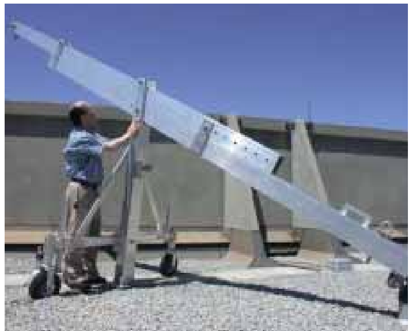
A portable outrigger (shown above) or davit may be used to avoid overloading a parapet wall.
