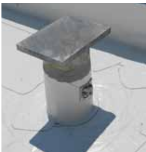
Standard davit pedestal; Compatible with Top Rotating or Ground Launched Davits
