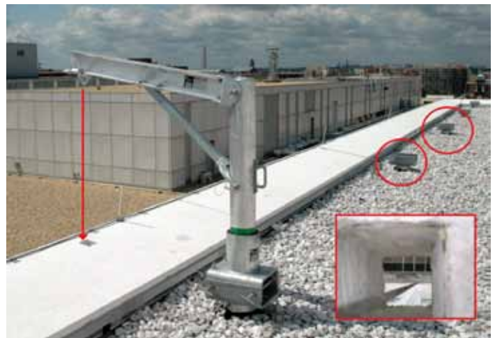
Davit pedestal bases were installed along the perimeter of this roof. The davit arm in the foreground can be moved to any davit pedestal base needed. Davits were installed to avoid loading the cornice. 5" x 5" sleeves were cast into the cornice to allow a suspended cable to pass through. This configuration maintains proper clearance between the suspended work platform and the façade.
