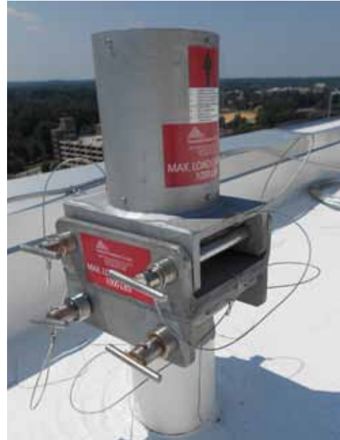
SM-DVT-SKT-P-* : Portable Davit Socket is attached to the top of the Davit Adaptor
