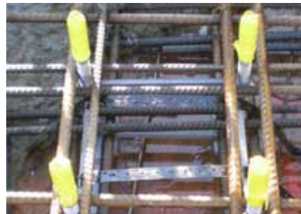
SM-DVT-CGE: Davit cage before and after pouring of concrete slab.
