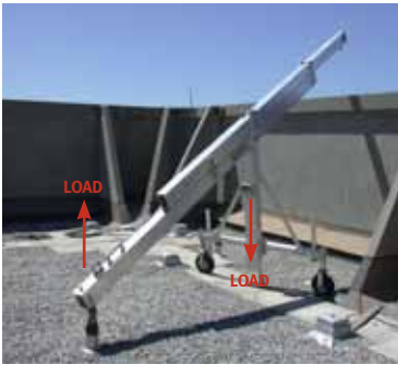
Left: A typical outrigger tied down to a single roof anchor. Unlike davits, outriggers do not concentrate their operating load into a single roof socket.
