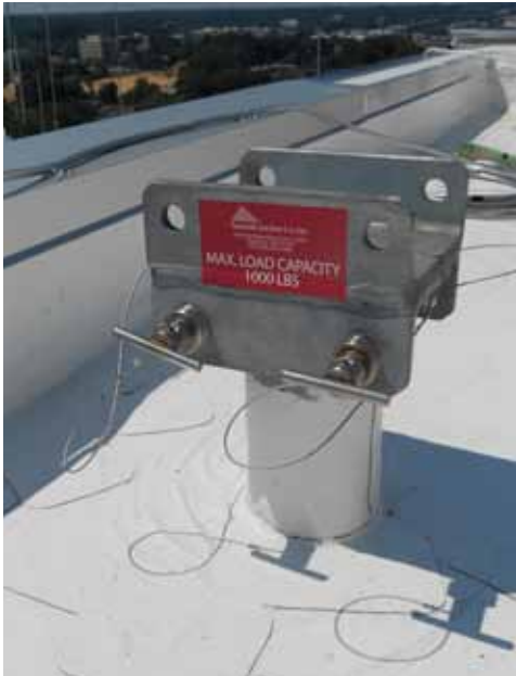
SM-DVT-PA-* : Portable Davit Adaptor is attached to the top of the Davit Pedestal
