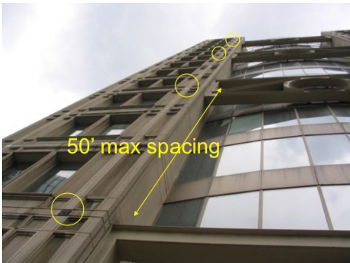
Single Intermittent Stabilization System with Anchor in Curtain Wall Mullion
