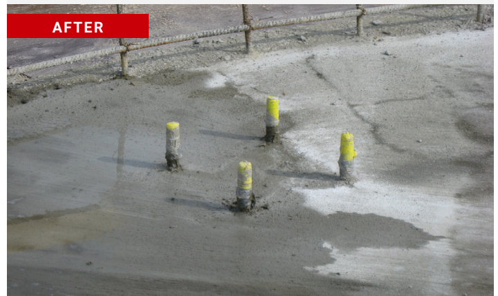
SM-DVT-CGE: Davit cage before and after pouring of concrete slab
