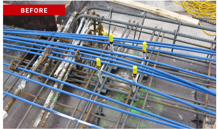
SM-DVT-CGE: Davit cage before and after pouring of concrete slab
