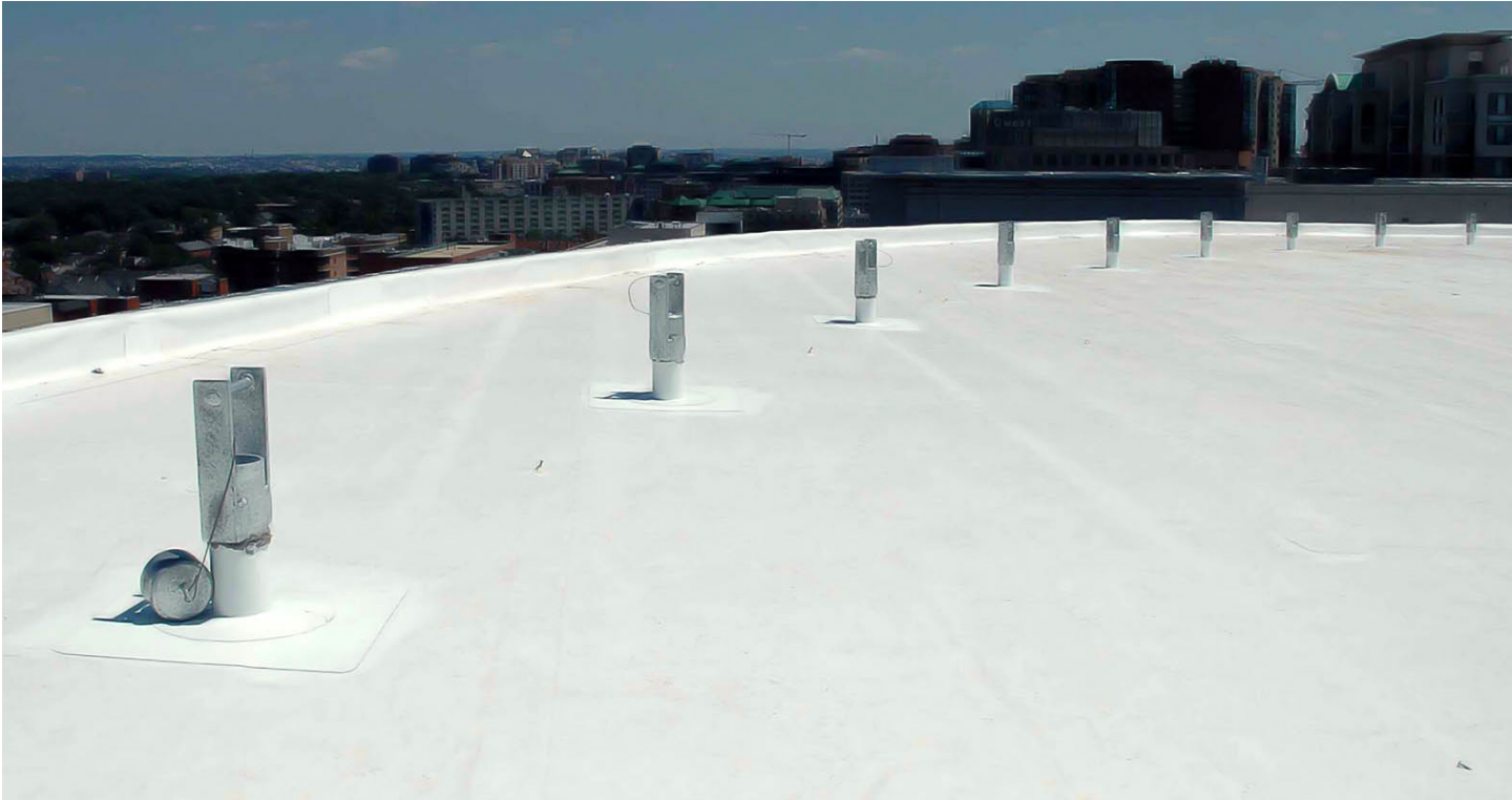
Rigging sleeves located on the roof above an overhang access to access the exterior facade shown on page 1 of this manual.
