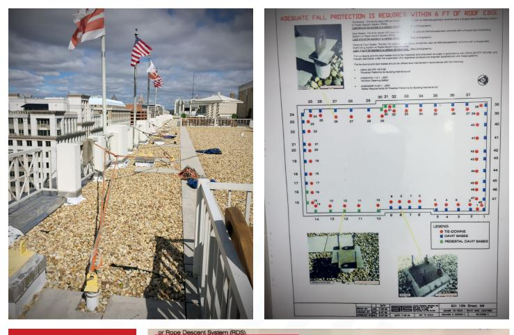
Load should be applied in a vertical direction only. (See photographs.)
