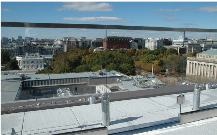
Figure 22 - HLL designed in conjunction with an access gate. Note that HLL was interrupted to reduce a trip hazard when walking through gate.
