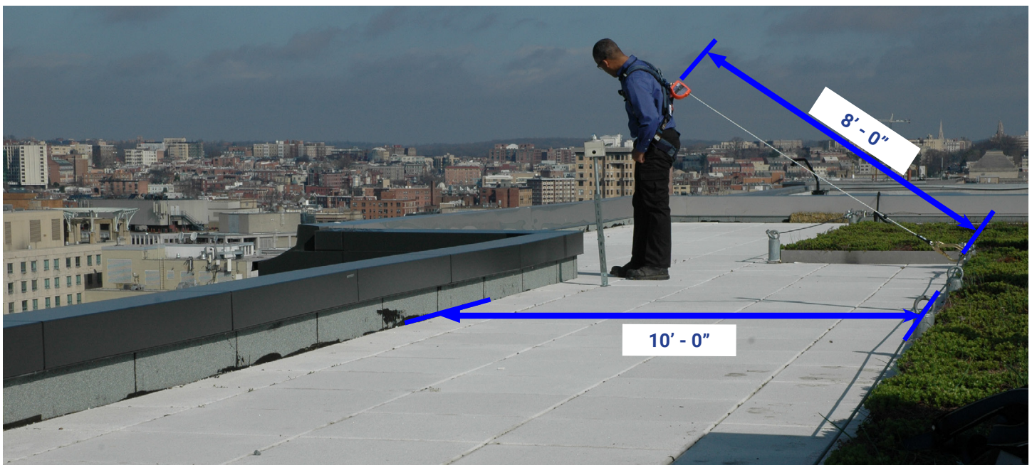
Figure 4 - Suggested placement of an anchorage with radius at building corner of fall restraint.
