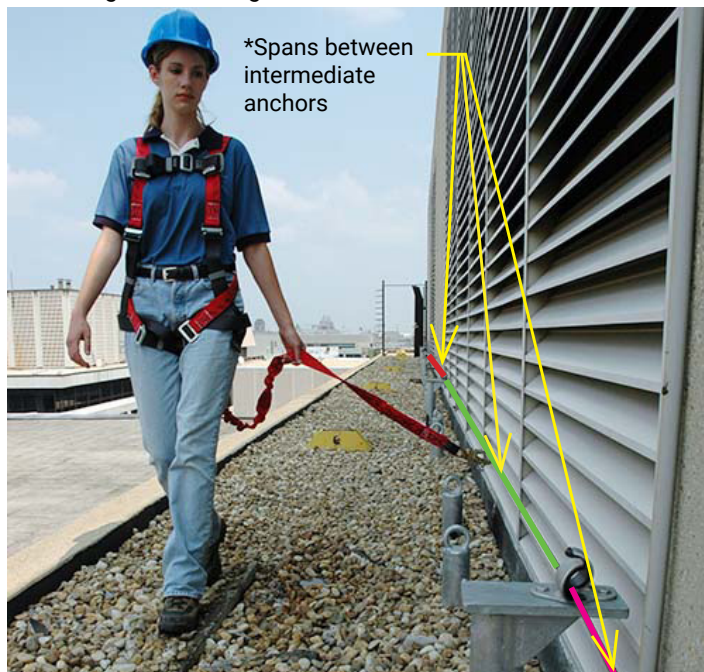
Figure 1: Worker using a horizontal cable system
