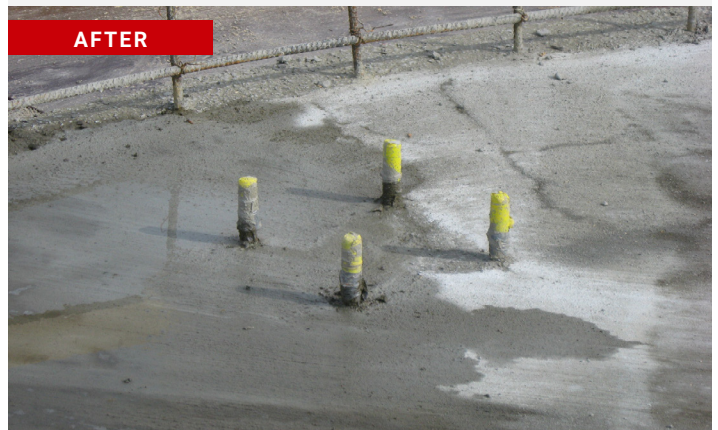
SM-DVT-CGE: Davit before and after pouring of concrete slab
