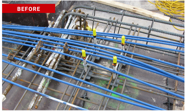
SM-DVT-CGE: Davit before and after pouring of concrete slab
