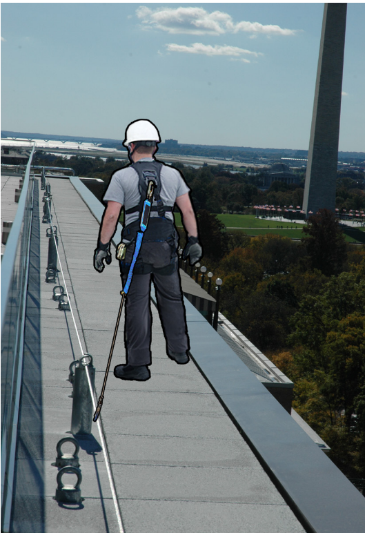
Figure 8 - Worker using a fall arrest system.
