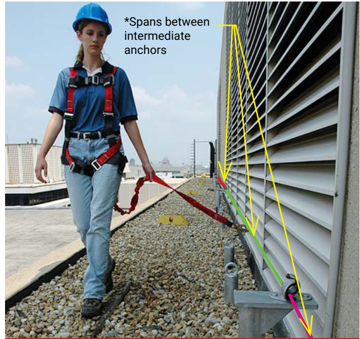
Figure 1: Worker using a horizontal cable system
