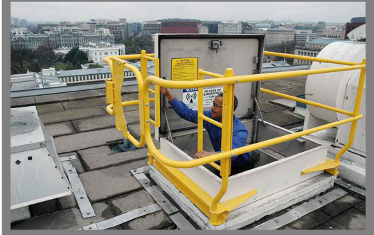
HATCH GUARDRAILS
