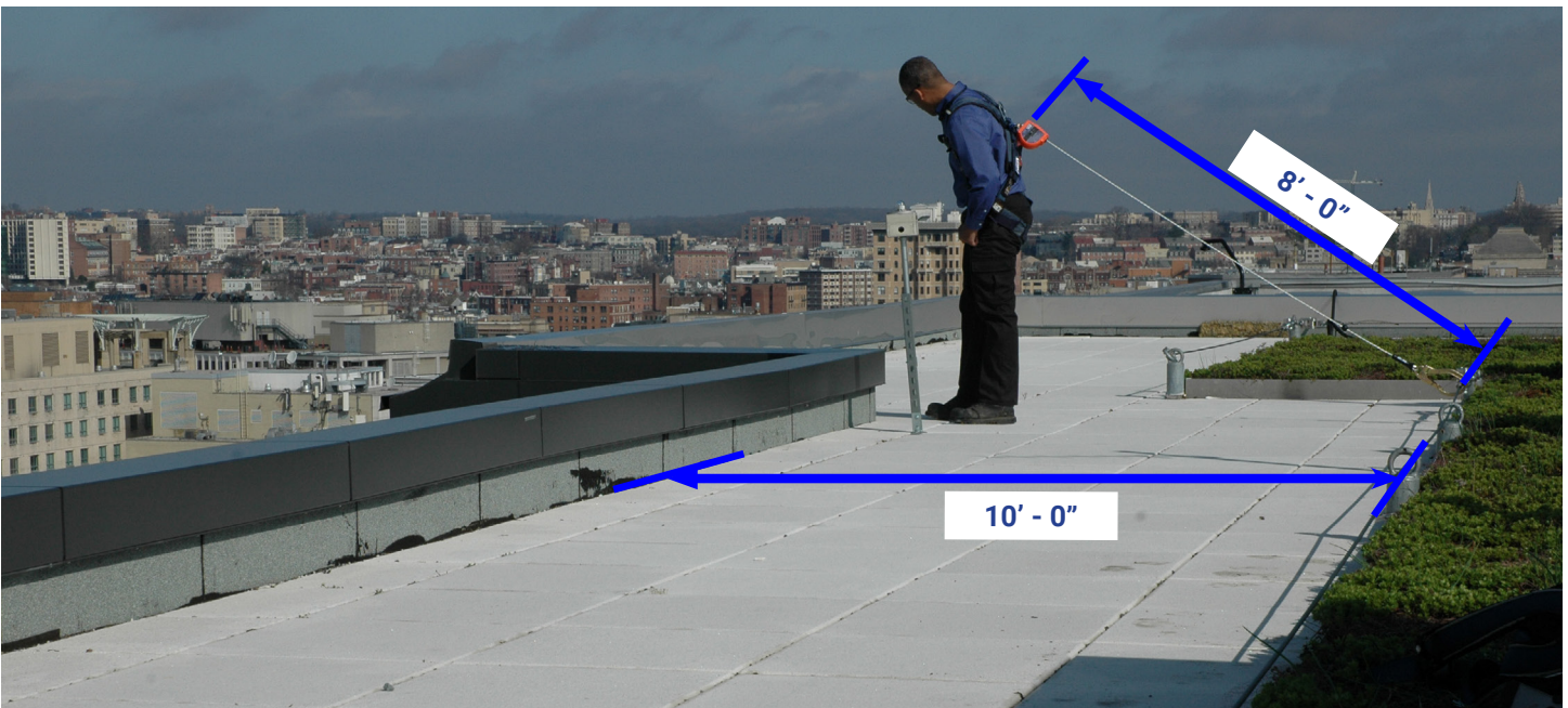
Figure 5 - Suggested placement of an anchorage with radius at building corner of fall restraint.
