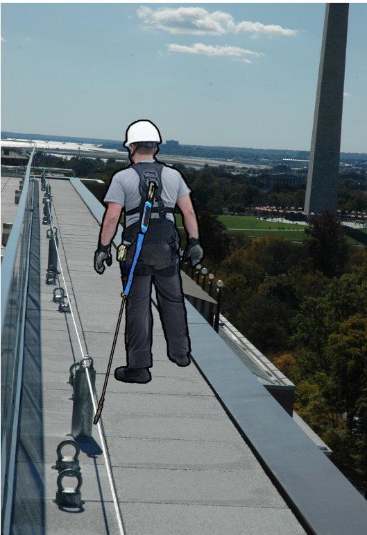
Figure 8 - Worker using a fall arrest system.
